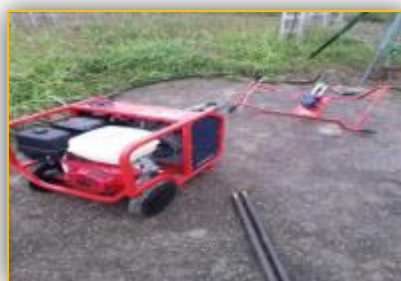
Figure 4. Motor drill "HYCON" in position for taking samples of contaminated soil, [1], [8] to [10]
